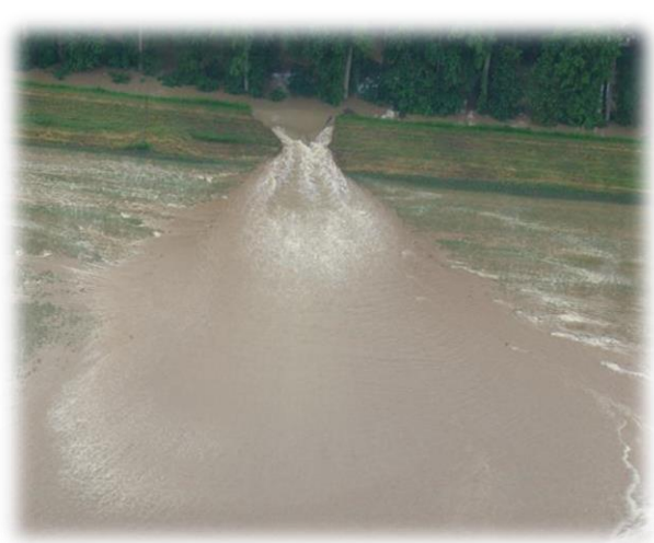
b) Embarrass River Dyke breach
