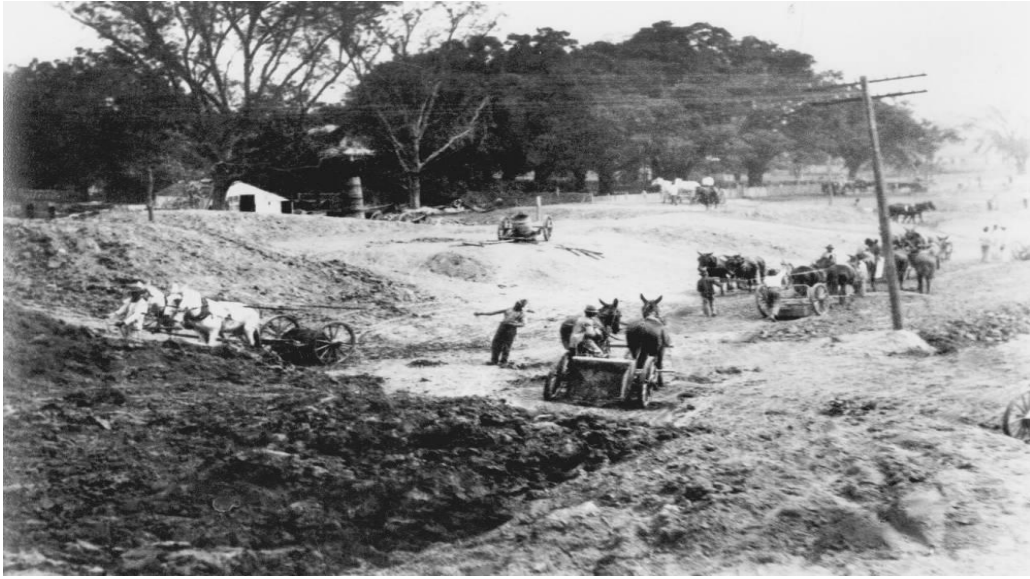
Figure 1.3 Early dyke constructions (ca. 1928) along Mississippi River (Courtesy U.S. Army Corps of Engineers)
