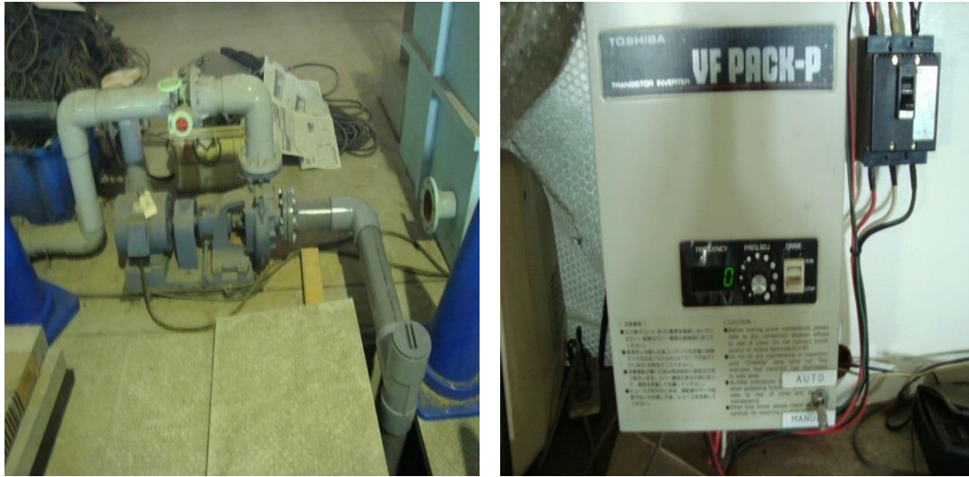
Figure 2.7 Pump arrangement and frequency controller
