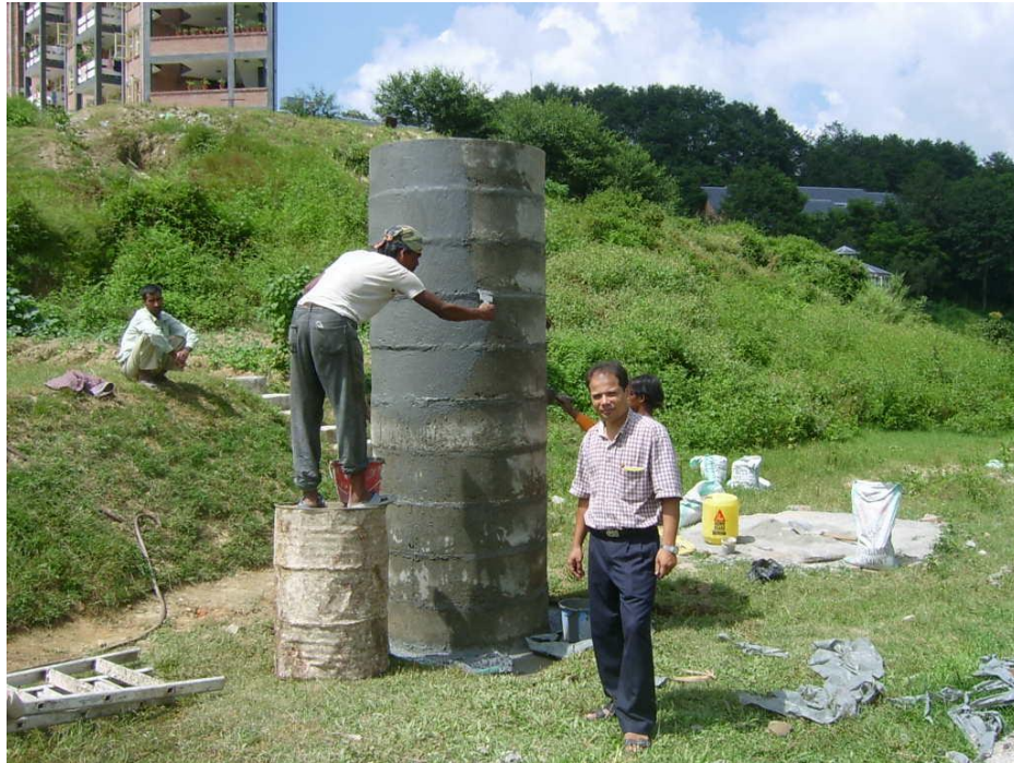
Photograph 9: Lysimeter Construction
