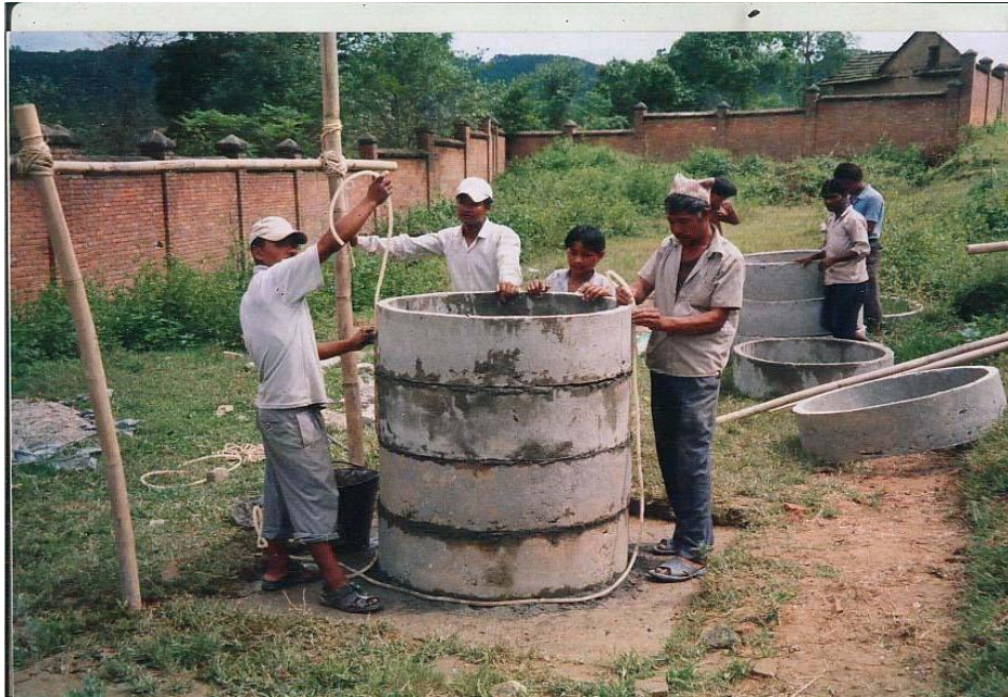
Photograph 3: Lysimeter Construction
