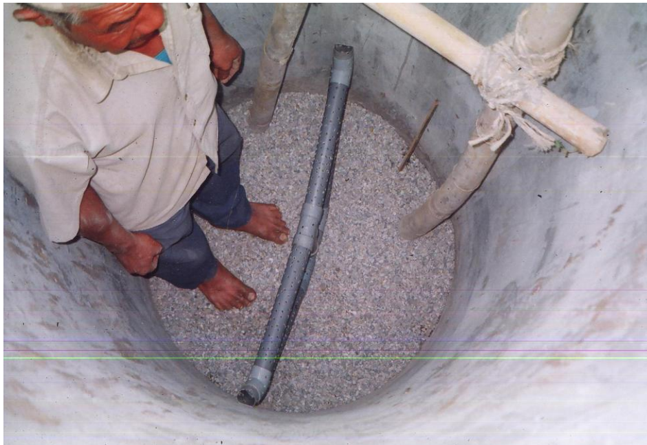
Photograph 10: Drainage Layer and PVC Pipe Fixation
