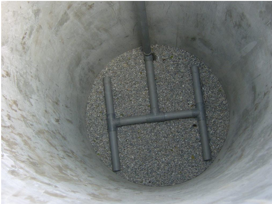
Photograph 6: Placement of Leachate Collection Pipes
