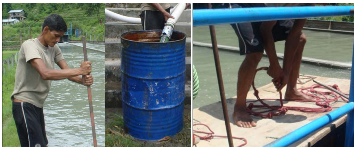
Figure 7-5: Measurement of sediment deposition level, discharge and relocation of suction head
