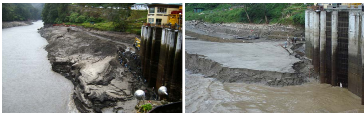
Figure 3-1: Sediment deposition in intake area of Chhukha HP (Chorten, 2010)
