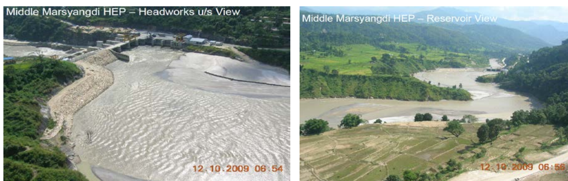
Figure 3-2: Sediment deposition in Middle Marsyangdi reservoir (Kayastha, 2010)
