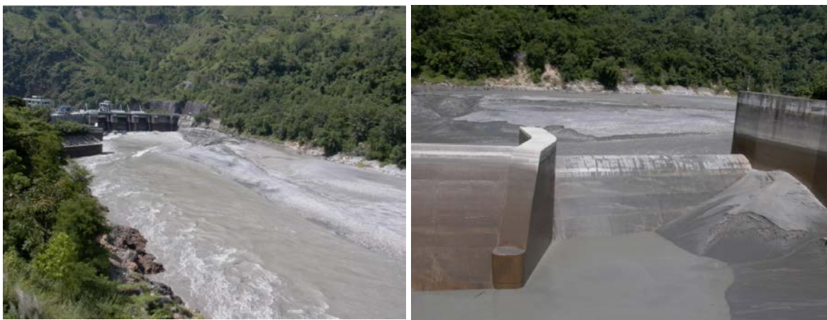
Figure 3-3: Sediment deposition in reservoir and forebay of Kaligandaki A reservoir during the flushing.
