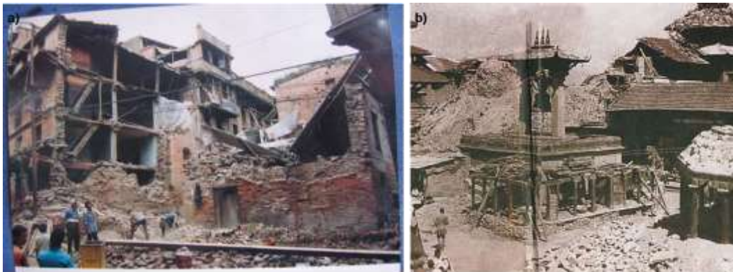
Figure 2.44: Typical example of a) buildings; and b) temples damage in Kathmandu Valley during 1934 earthquake.
