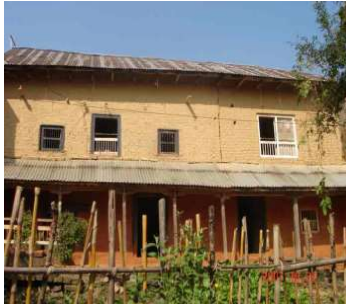
Figure 7.1: An example of Adobe building.
