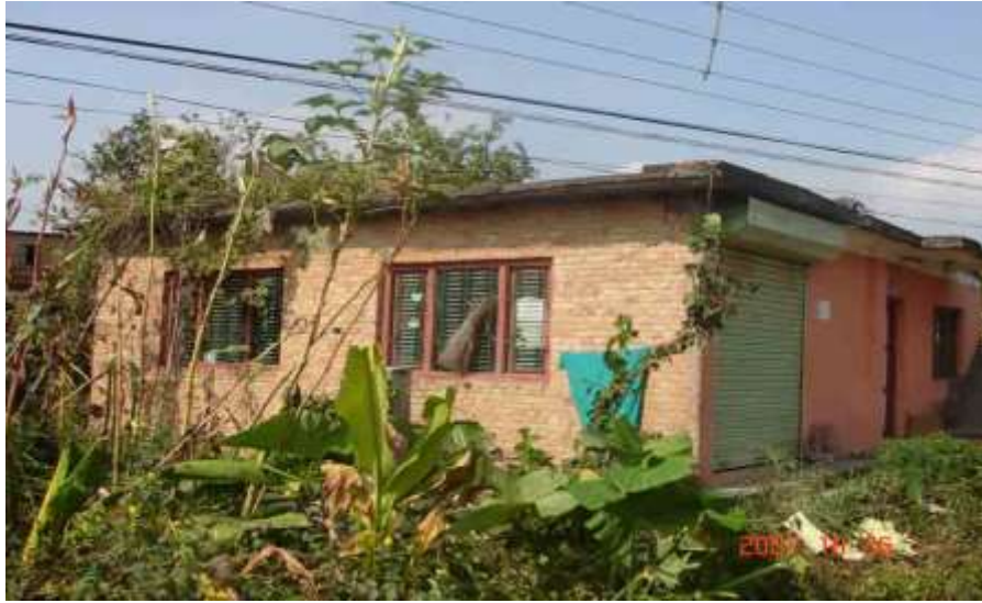
Figure 7.3: An example of BM building.
